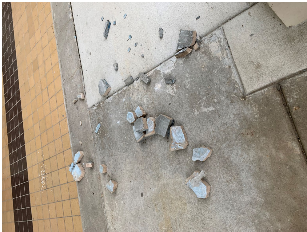
CRUMBLING CONCRETE – February 2020
