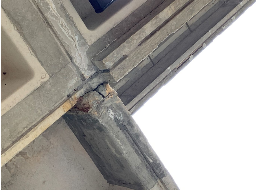
LOOSE OVERHEAD CONCRETE – February 2020
