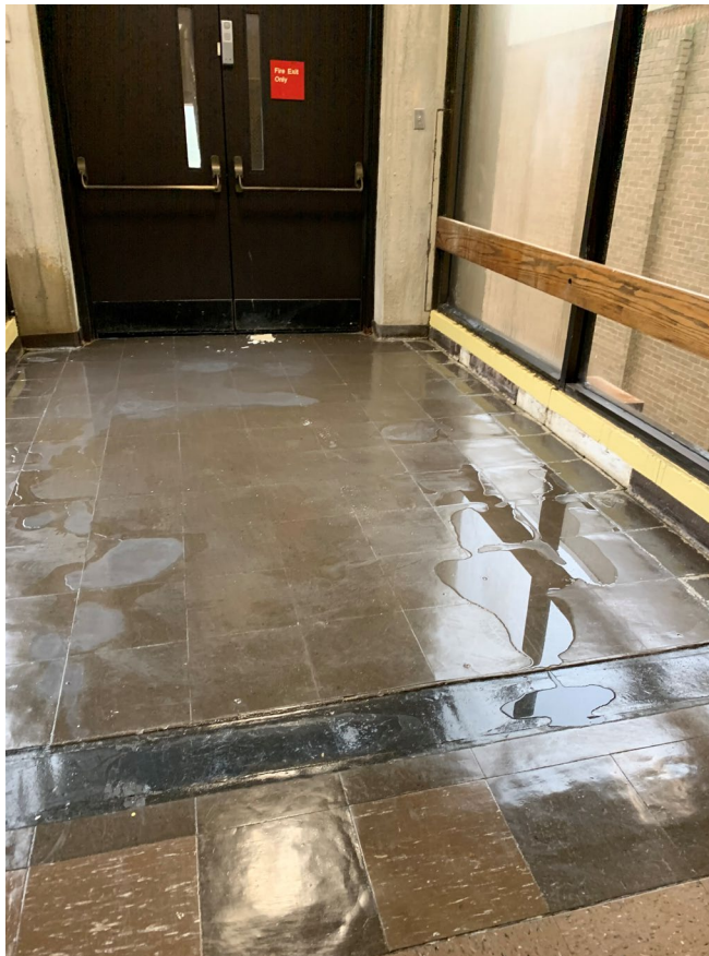
WATER INTRUSION AT STAIR TOWERS – February 2020
